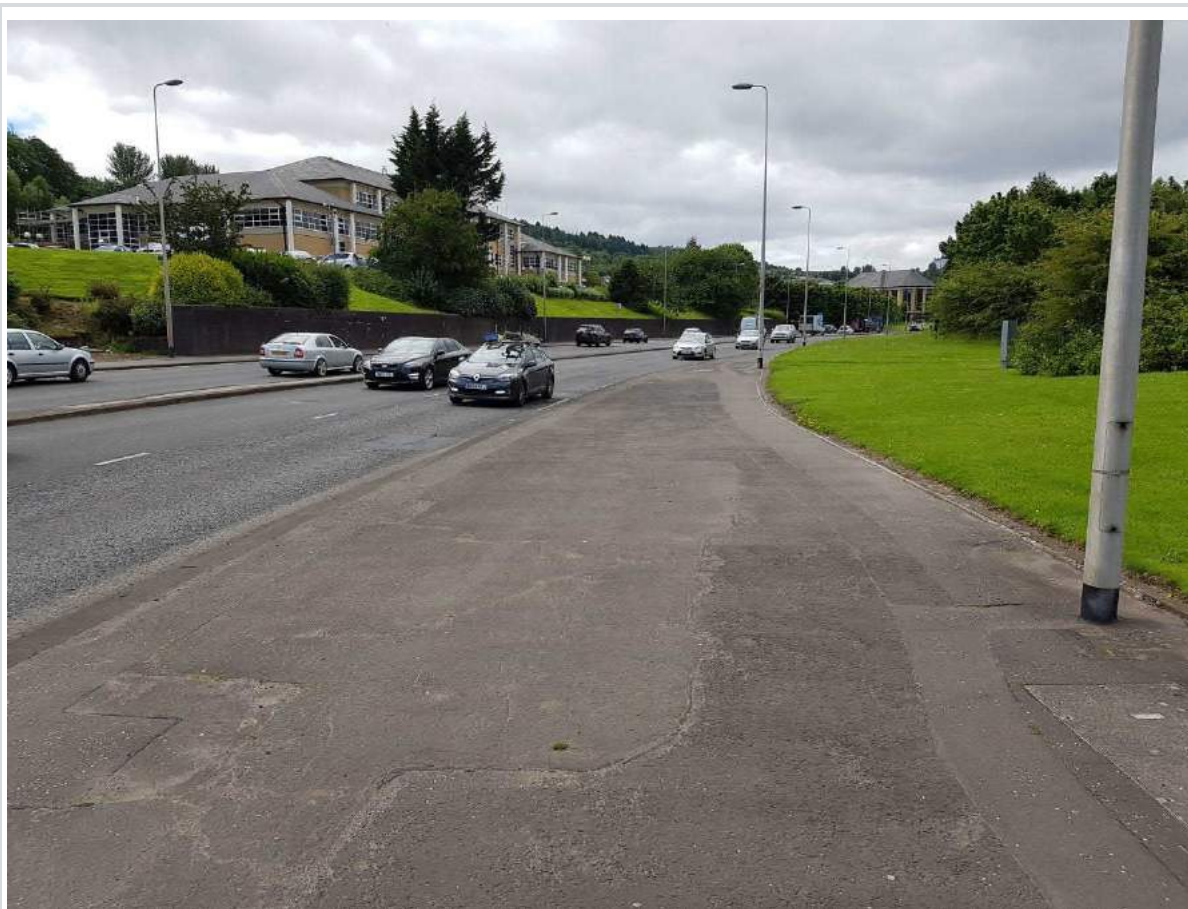
Figure 3.4: A8 (T) Footway
