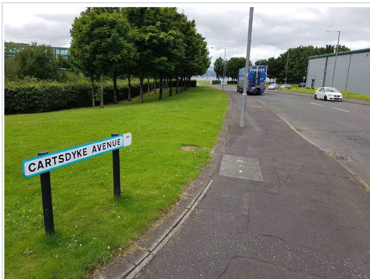
Figure 3.2: Existing footpath on Carttsyke Avenue
