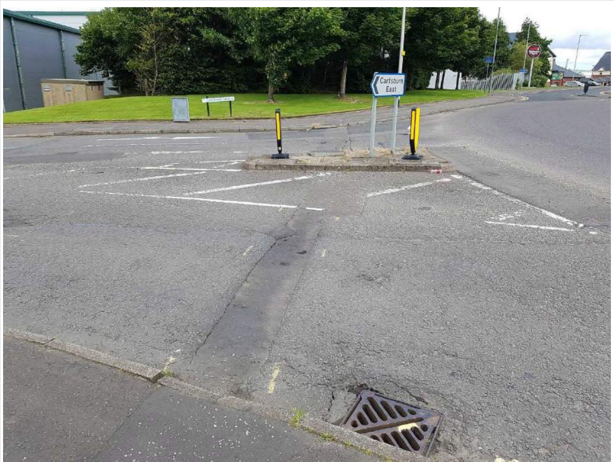
Figure 3.3: Arm of Cartsdyke Avenue and Refuge Island
